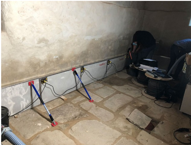
The FastDry system in use in the historical bathhouse.
