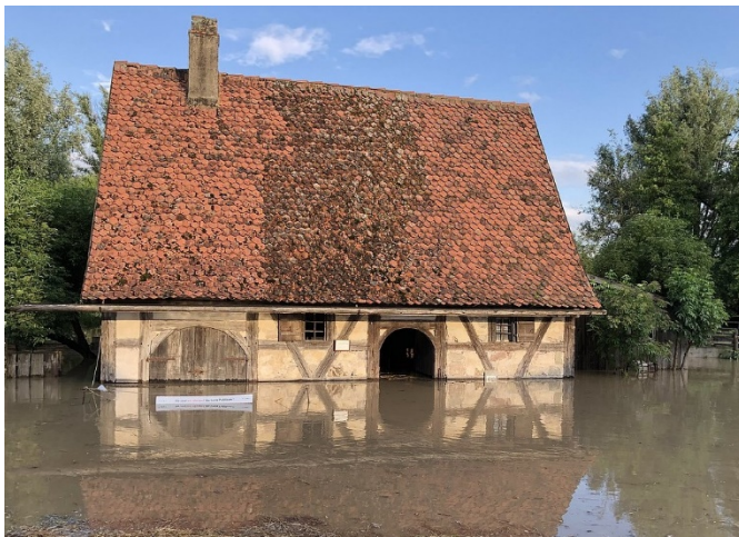
Historical buildings affected by the Aisch flood disaster in July 2021.
