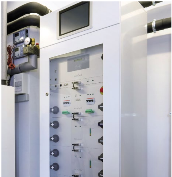
Battery storage, 13.2 kilowatt hours
