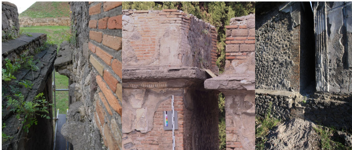
Fig. 8: damaged cornice PN_EN_4, 6_DSC_0426
