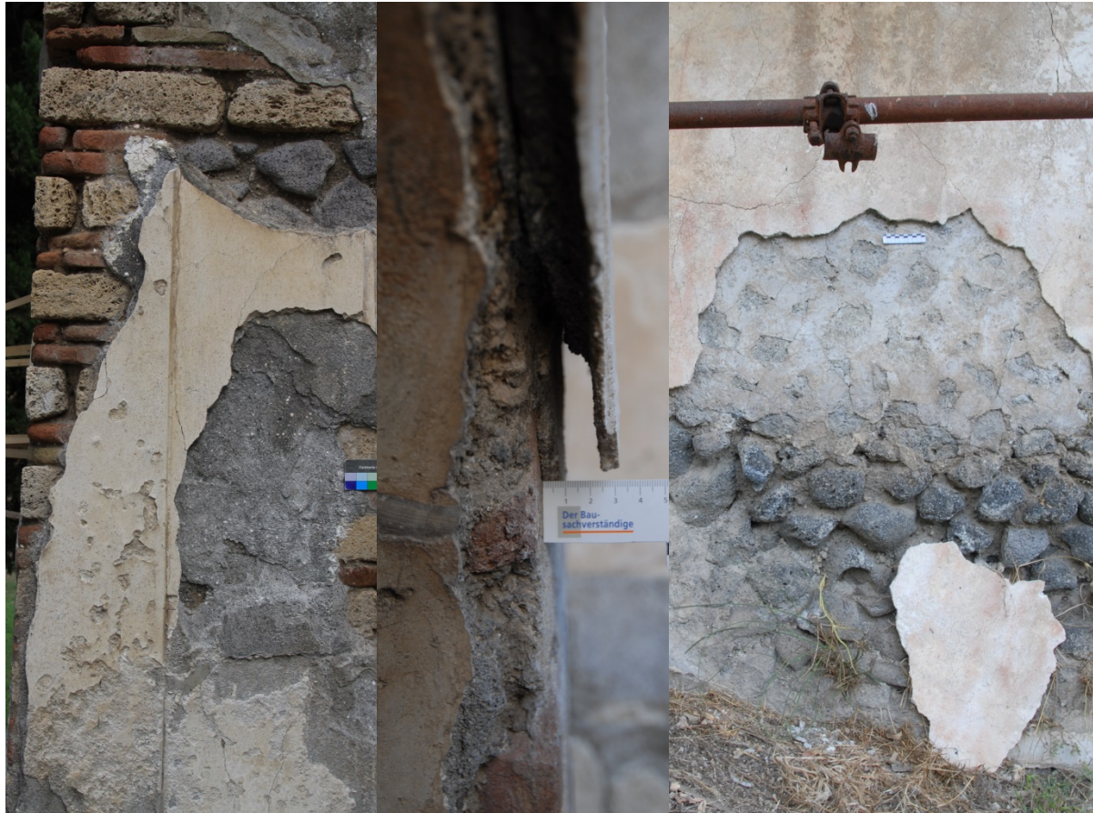
Fig. 9: damaged plaster PN_EN_12_S_IMG_4230
