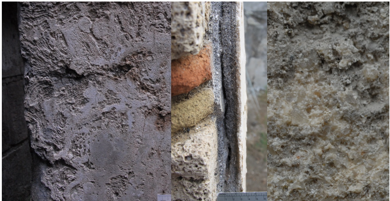
Fig. 11: Deterioration by humidity & salts Pn_OS_29_S_DSC_0351 PN_EN_12_S_IMG_4229 PN_EN_12_S_DSC_0254
