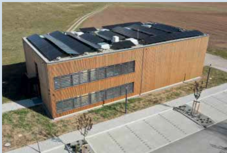
Figure 58: PV system on the roof of the hall Photograph: City of Feuchtwangen
