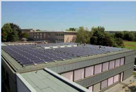
Figure 46: PV system on the roof of the new build Photograph: Town of Kaufbeuren
