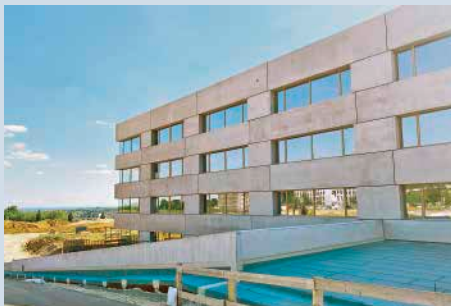
Figure 78: East side of the building Photograph: SPREEN ARCHITEKTEN
