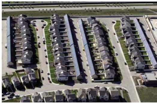
Figure 7.19: Okotoks complex (Canada).
