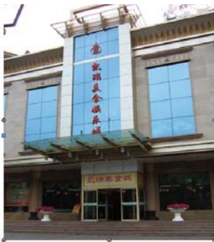
Shihezi Kai Rui Building
